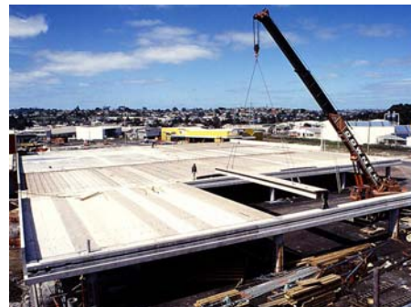
Rapid placement for large areas
