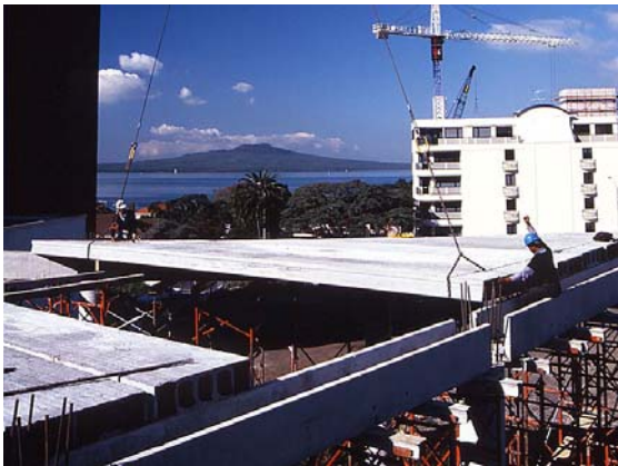
Cor slab on shell beams
